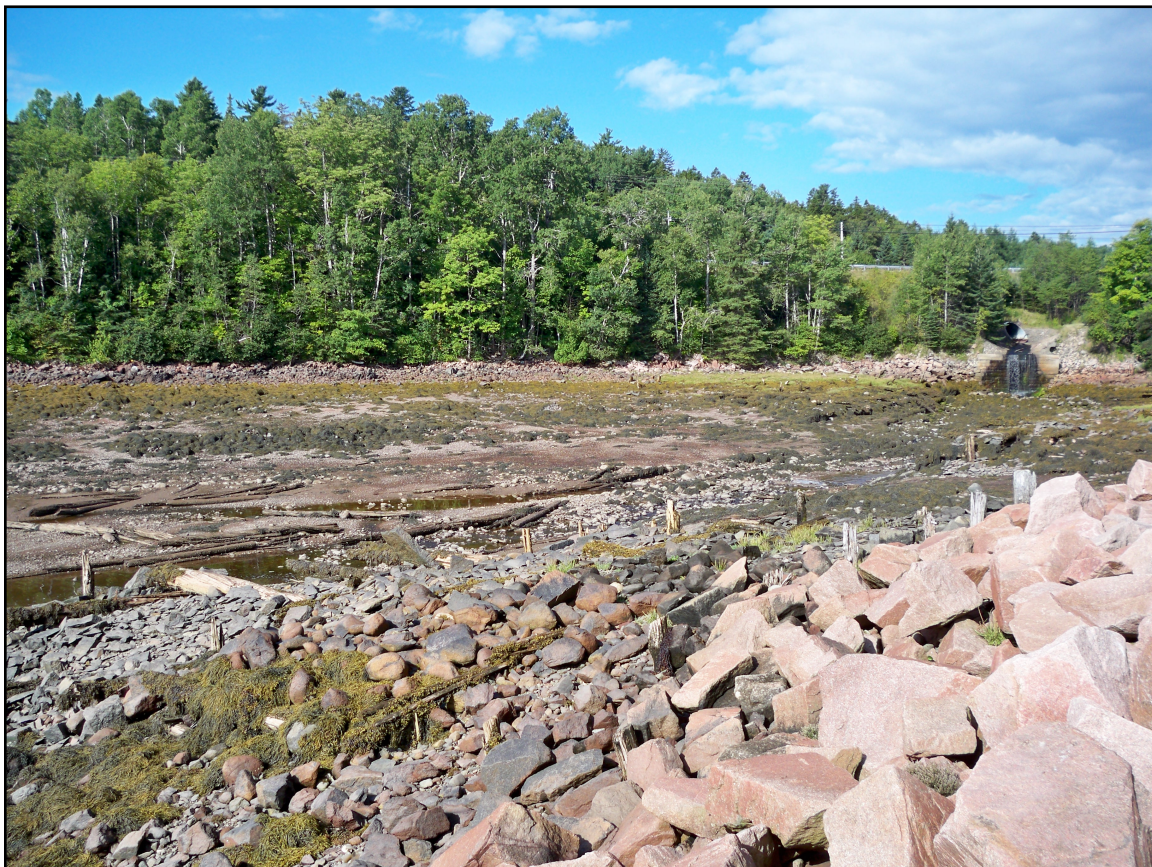
Figure 4.12. Historic Structures at Red Beach Cove (Mather 2010)
